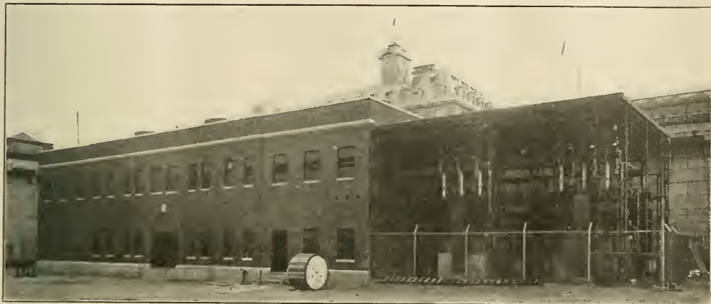
Exterior of St. George Substation
